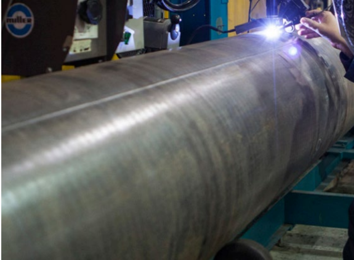
Photo 61: BBVC Case Welds
